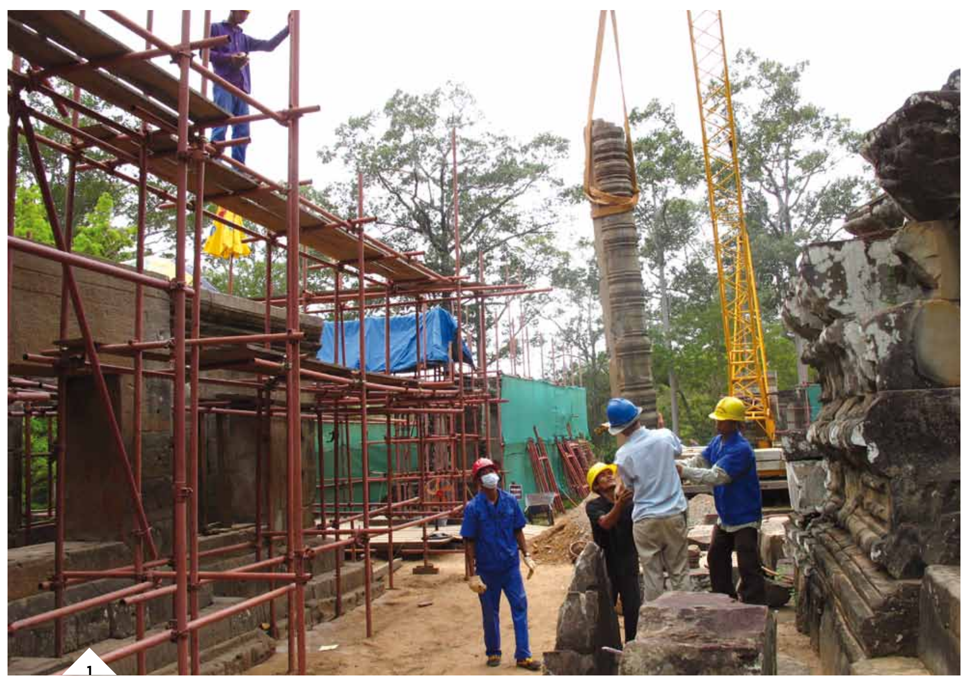
▲ 1. Assembling a colonette on southern interior gopura ▲ 2. Putting stone components back to original positions at eastern exterior gopura ▲ 3. Laser scanning of Takeo temple (GEOLAB) ▲ 4. Dismantling process of corner tower of southwest corner, second tier platform
